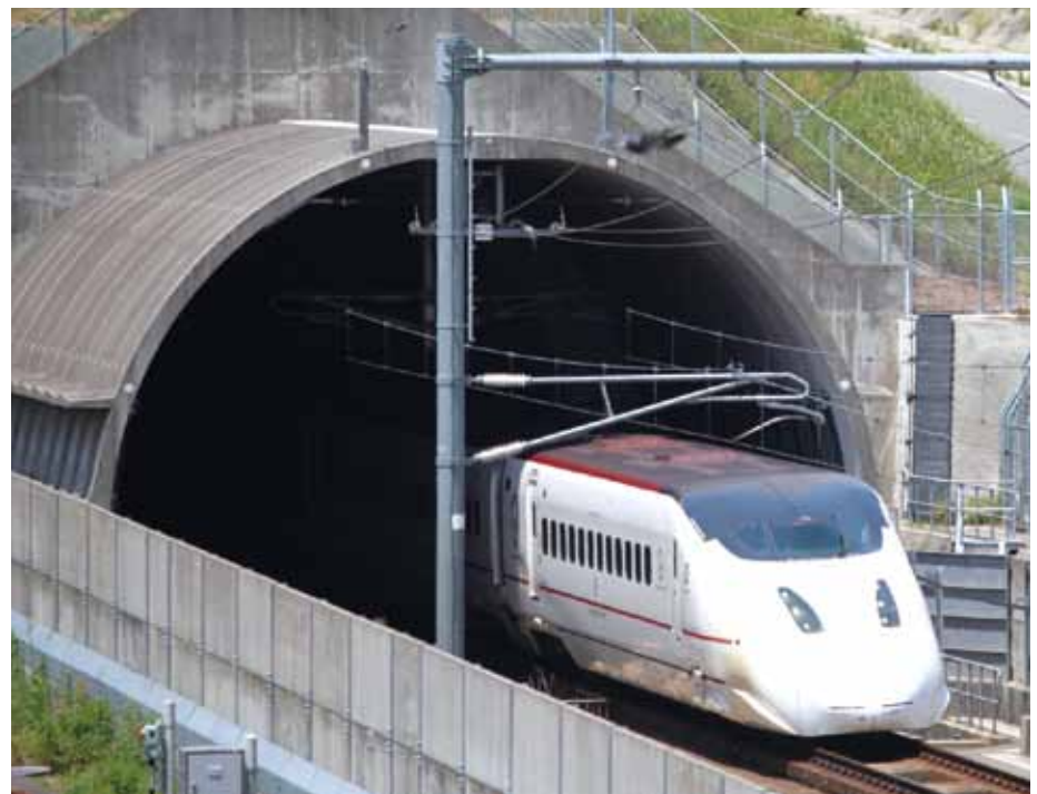
Tunnel entrance hood
