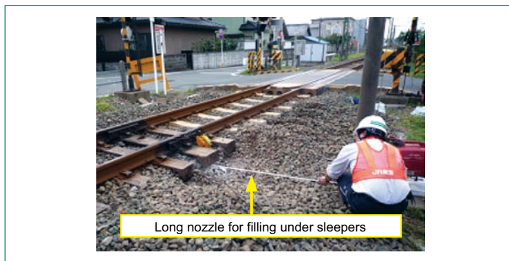
Fig. 16 Filling work using air pressure
