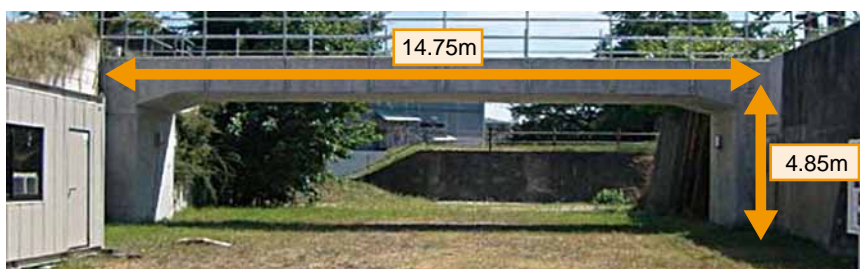
► Full scale mock up of reinforced embankment jointless bridge
