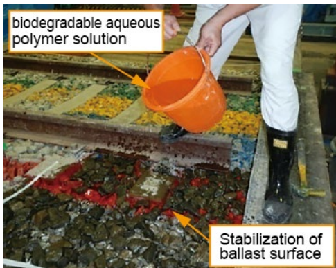
Fig 3 Stabilization of ballast using polymer solution
