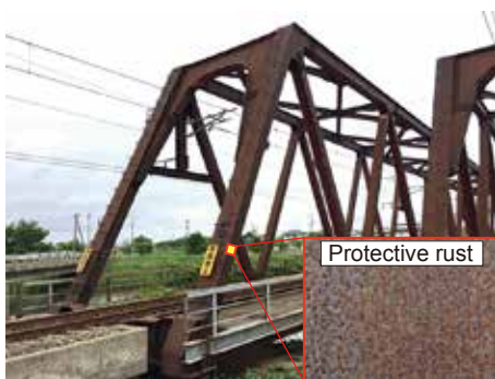
Fig. 1 Weathering steel bridge
