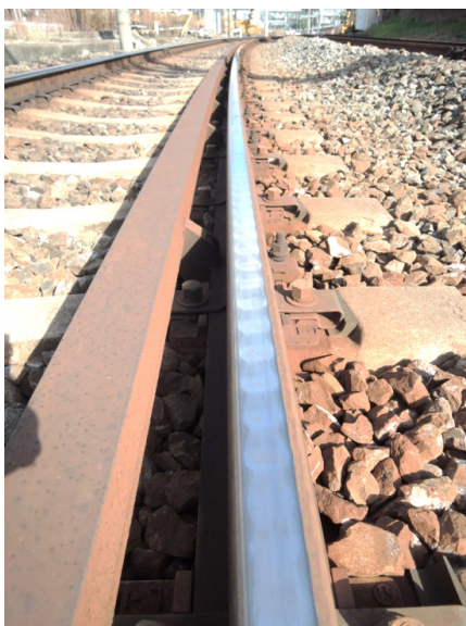
Fig. 1: Example of rail corrugation generated on a curve
