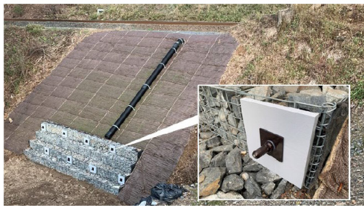
(a) View of the repaired embankment
