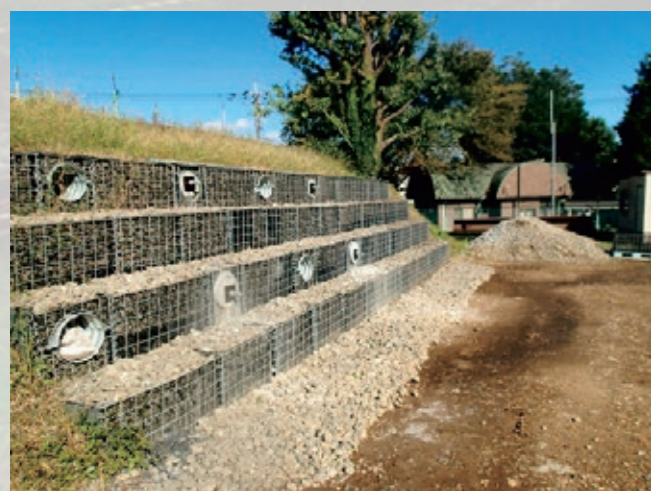
地震・豪雨等による被災盛土の早期・強化復旧技術 Quick repair and reinforcement method for embankments damaged by earthquakes and rainfall
