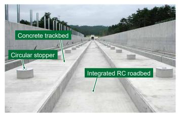
Integrated RC roadbed (Before a track slab is laid)
