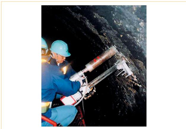
**Fig. 1** Obtaining concrete samples
