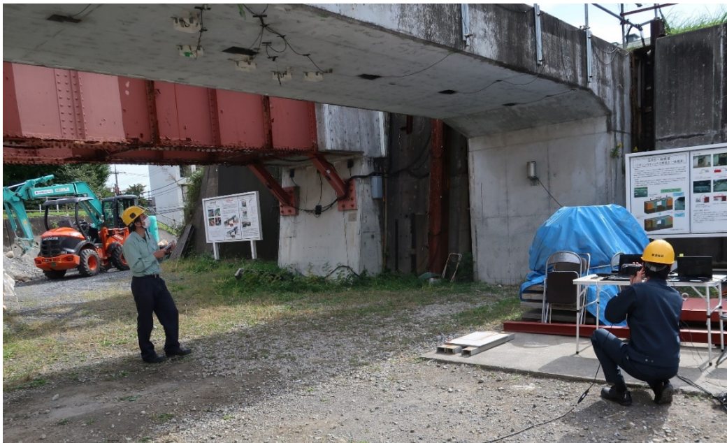
Live streaming from the test field reproducing railway structures at RTRI Visual inspection support system using 3-dimensional images
