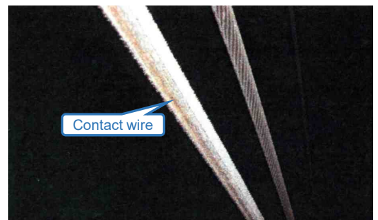
Fig.2 Frost formation on the contact wire
