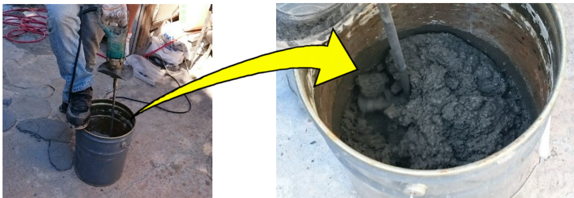
Fig. 4 Preparing geopolymer mortar with handheld mixer
