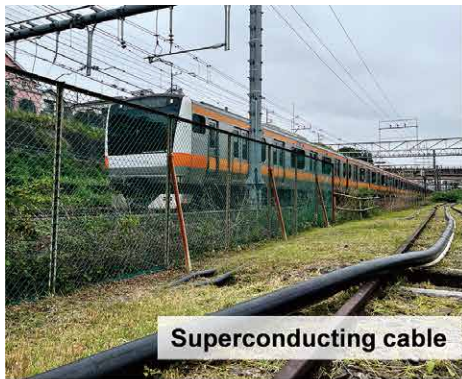
Fig. 4 Train running through a power supply section consisting of the superconducting feeding system (high-current power supply on the JR East Chuo Line)
