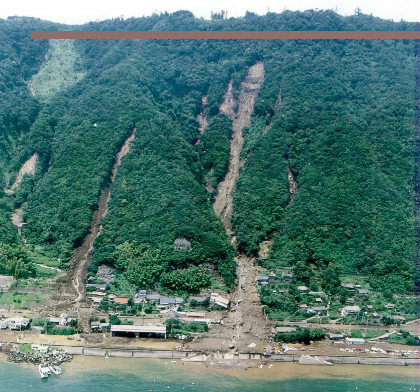
Figure 1 Debris-flow event that occurred near Ryugamizu Station on the Nippo Main Line in August 1993 1) (trimmed)
