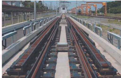
Figure 2. Gauge-changing device.
