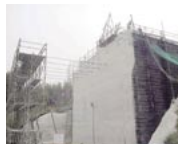
Figure 6. View of the lateral loading test in Kyushu.
