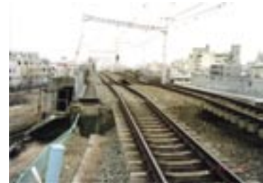
Figure 2. A damaged bridge abutment at Hyogoken-Nambu Earthquake (January 17, 1995).
