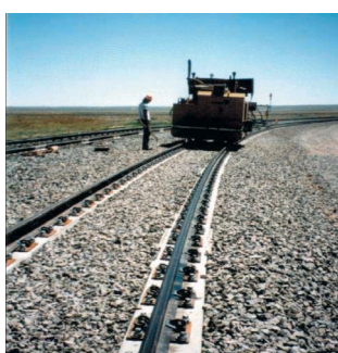
Figure 3. Ballasted ladder track in TTCI.
