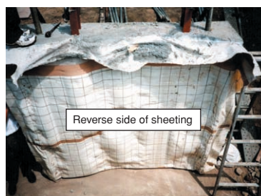
Figure 4. Adhesive waterproof sheeting bonded to concrete
