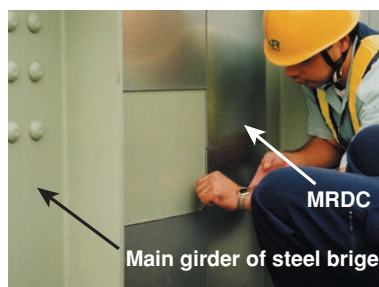
Figure 3. A picture of installation of MRDC.
