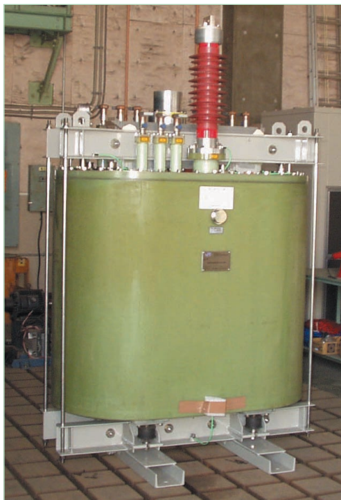
Figure 1. Appearance of the test-manufactured superconducting main transformer
