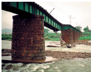
Fig. 1 Destructive effect of scouring under a railway bridge (Japan)
