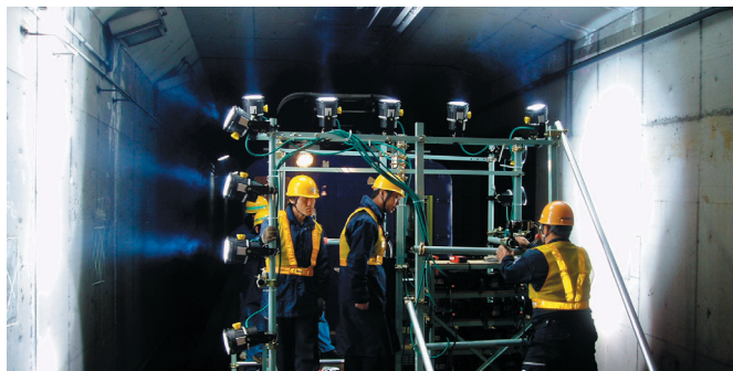
Fig.1. Tunnel-scanner system for tunnel wall image recording.
