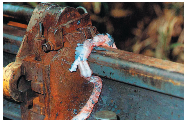
Fig. 3 Hot shearing method being used to remove a bulge
