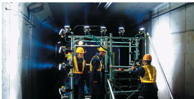
Fig. 1. Tunnel-scanner system for tunnel wall image recording.
