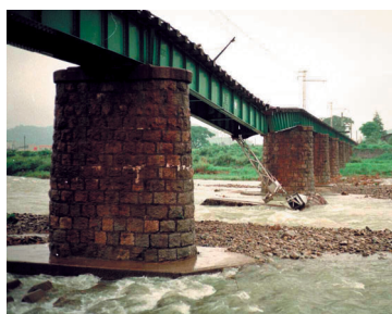
Fig. 1 Destructive effect of scouring under a railway bridge (Japan)
