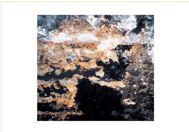
**Fig. 2** Concrete surface deterioration due to acidification
