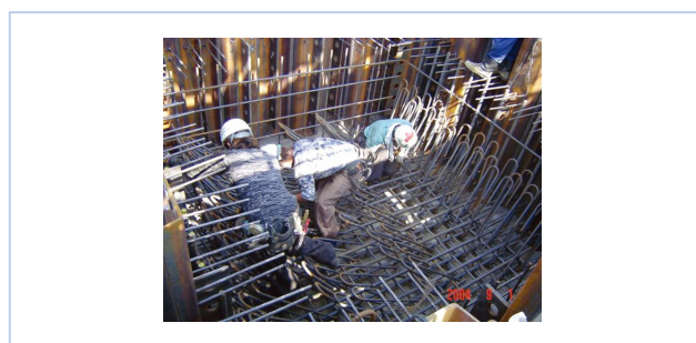
Fig. 2 Assembly of footing reinforcing bars
