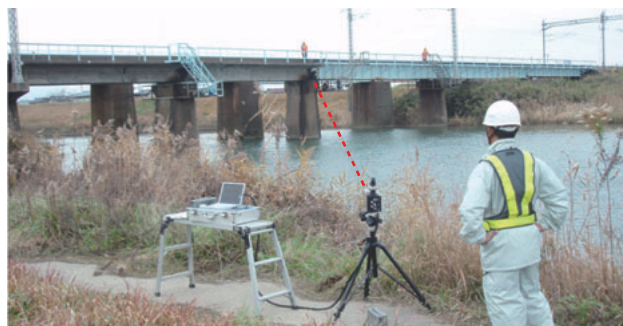
Fig. 2 Measurement of bridge pier vibration by U-Doppler
