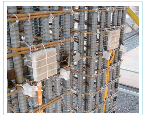
Fig. 5 Installation of sensors
