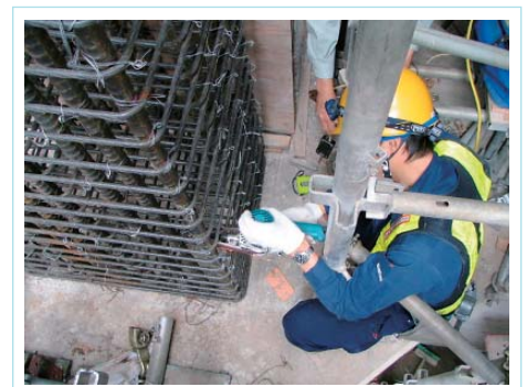
Fig. 4 Installation of detection sensors (to collect data from a rigid-frame viaduct)
