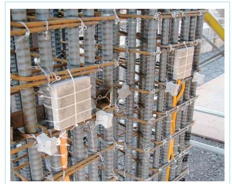
Fig. 5 Installation of sensors
