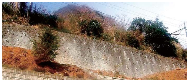
Fig. 4 Appearance of reinforced masonry wall
