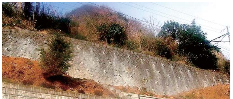
Fig. 4 Appearance of reinforced masonry wall
