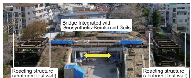
Fig. 2 Alternating horizontal loading test set up
