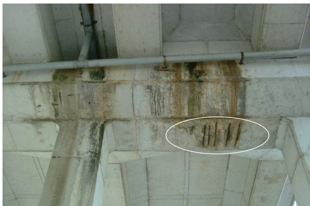
Fig.1 Exposed rebars where water splashes
