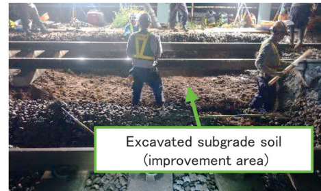
(a) Excavation of subgrade soil
