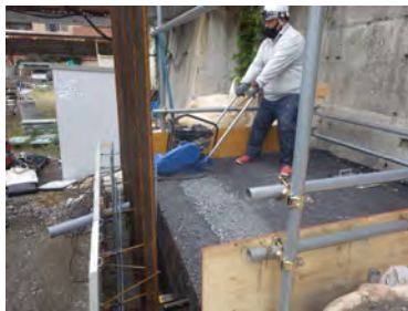
④補強盛土構築
