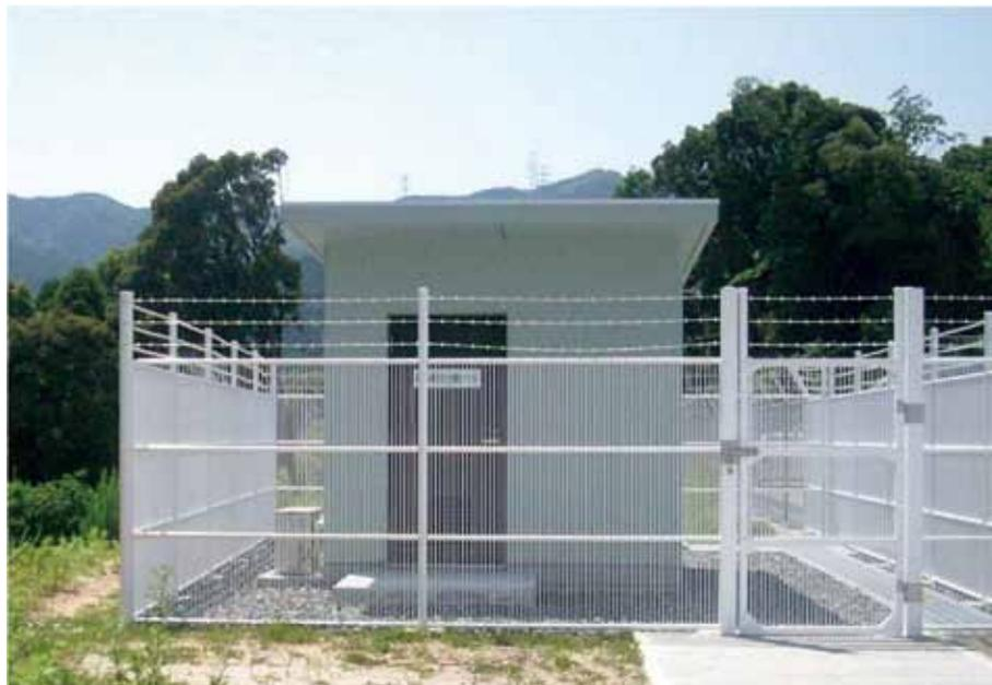
Detection points are located along railway tracks or quiet places distant from tracks. Constant temperature and humidity are maintained inside the buildings housing seismometers in order to ensure stable operation of the seismometers over a long period.
