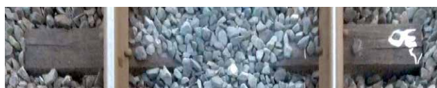
Figure 3 Standard for evaluating deterioration levels of wooden sleepers
