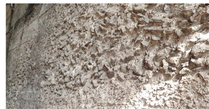
Fig. 21 Unevenness of lining
