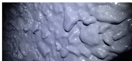
Fig. 24 Condition of surface of lining after spraying
