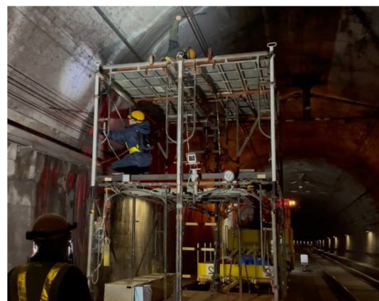
Fig. 2 Hammer sounding inspection along tunnel lining
