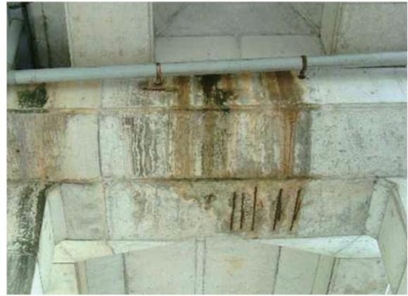
Fig. 2 Supplied water and spalling of concrete [3]
