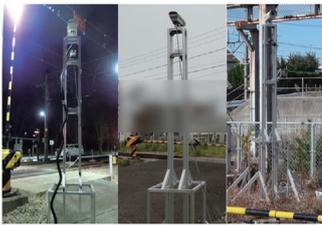
**Fig. 9 Temporary installation of cameras at level crossing in training facilities**
