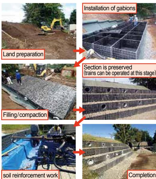
Fig. 1 Proposed construction work flow
