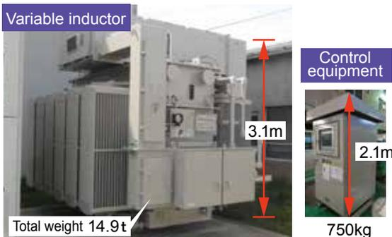
Fig. 1 Prototype voltage control equipment
