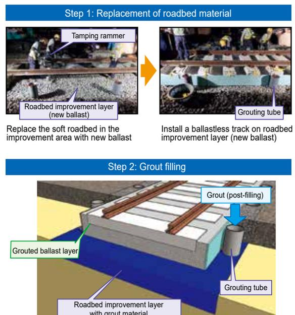
Fig. 2 Post-filling roadbed improvement method
