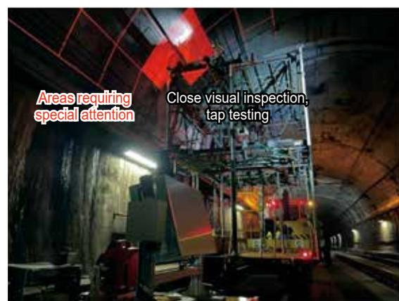
Figure 3 Inspection situation while projecting
