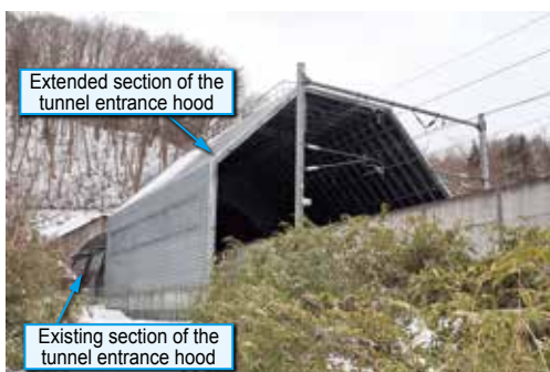
Figure 3 Two-step cross-sectional tunnel entrance hood installed in a Shinkansen tunnel
