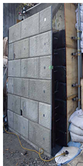
Lightweight buried formwork (Construction process viewed from the rear side)
