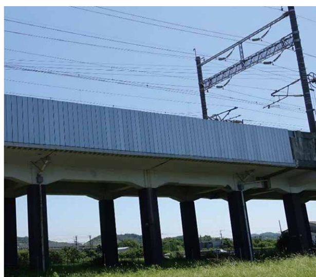
Installation example of modular noise barrier
