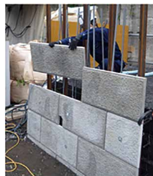
Lightweight buried formwork (Construction process viewed from the rear side)
