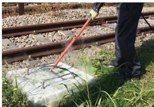
Example of practical application of steam weeding equipment
