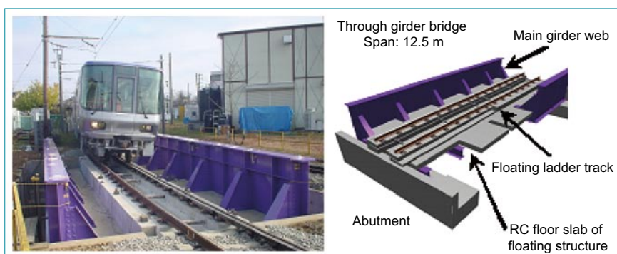
A new type of steel bridge with a floating structure
